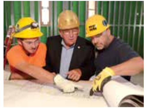
April 2016, Walsh begins construction of the new Global Learning Center.
